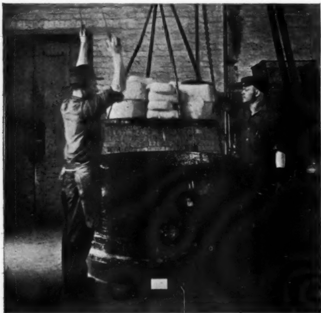
Impregnating a Lot of Field Coils
